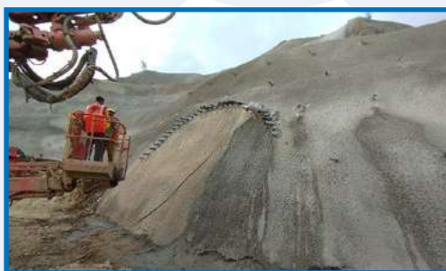
Fig 2: Opening of new face for tunnel after portal stabilization
