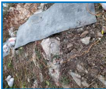
Fig 5: Successfully crack generation with minimum throw of the material after blast
