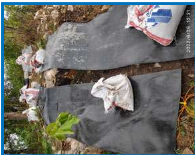
Fig 4: Trail blast with muffling of face
