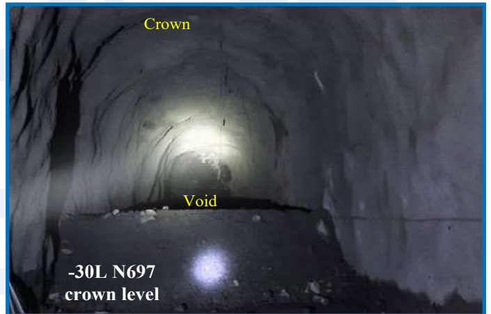
Fig. 19: Investigation of the crown pillar of paste fill material at underground in RAM, HZL.
