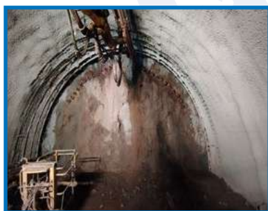
Fig 1: Face advancing with pipe roofing at BBB
